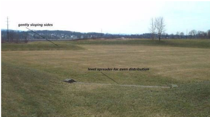
Figure 9-12. Level spreader distributes stormwater into the infiltration basin.
