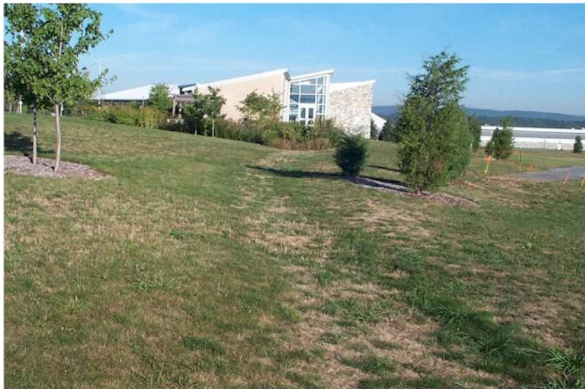
Figure 9-4. Infiltration trench located on contour, State College, Centre County.
