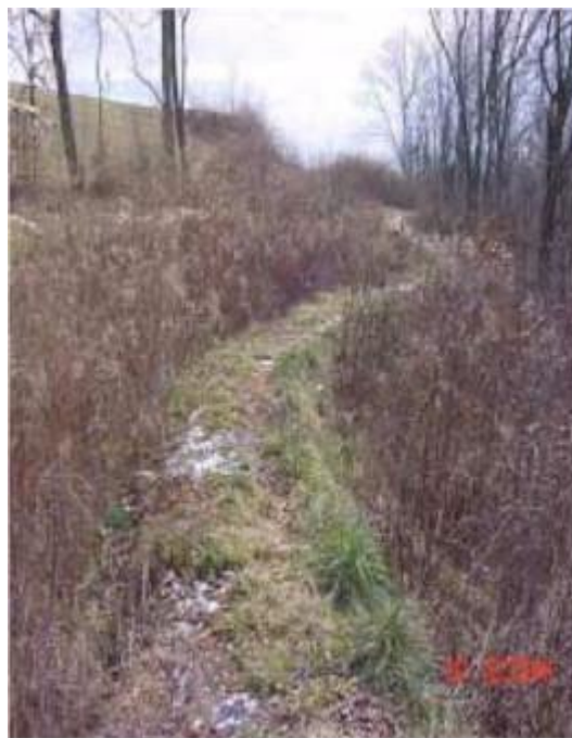
Figure 9-33. This grassy path is an embankment, or berm, creating depressions for recharge trenches located to the left of the path.
