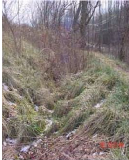
Figure 9-34. Narrow, vegetated infiltration trenches/berms follow land contours and take on a naturalized appearance.
