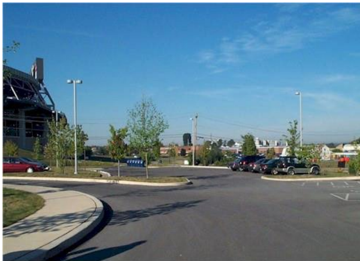
Figure 9-6. Porous asphalt parking lot, State College, Centre County.
