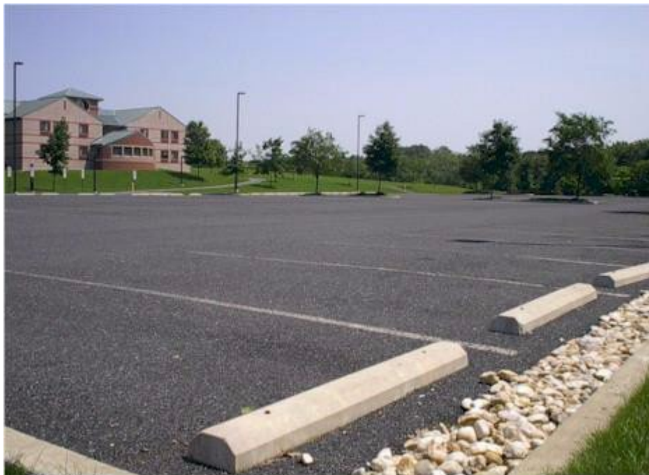
Figure 9-29. Porous asphalt parking lot with subsurface infiltration bed.
