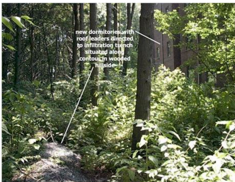
Figure 9-27. Level spreader pipe/infiltration trench in woods.
