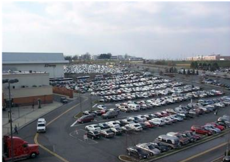
Figure 2-2. Parking lots are common impervious surfaces that affect stormwater runoff.
