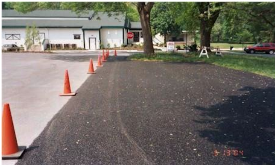
Figure 9-23. Completed porous asphalt parking lot at Ephrata Performing Arts Center.
