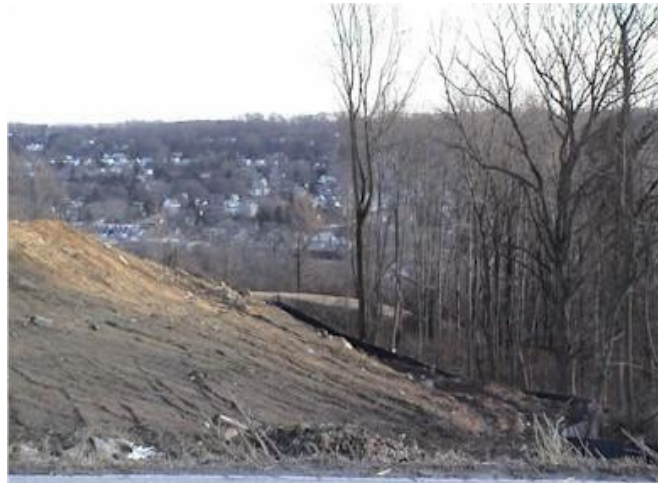
Figure 5.1-4. Steep slope development with woodland removal.
