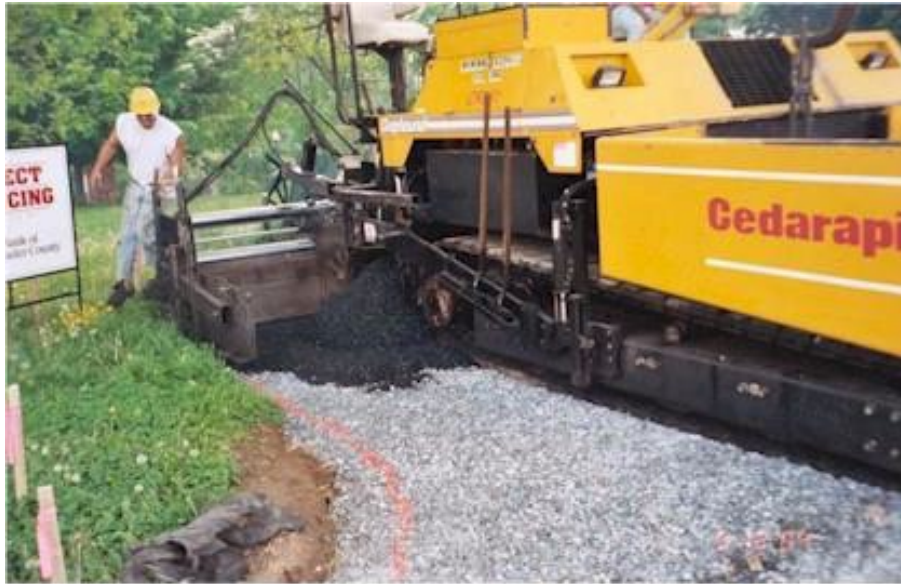
Figure 9-22. Construction of porous asphalt parking area to compliment building expansion.
