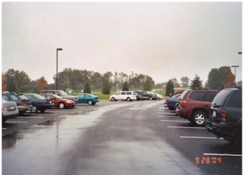
Figure 9-24. Completed porous asphalt parking lot at Lebanon County Conservation District.
