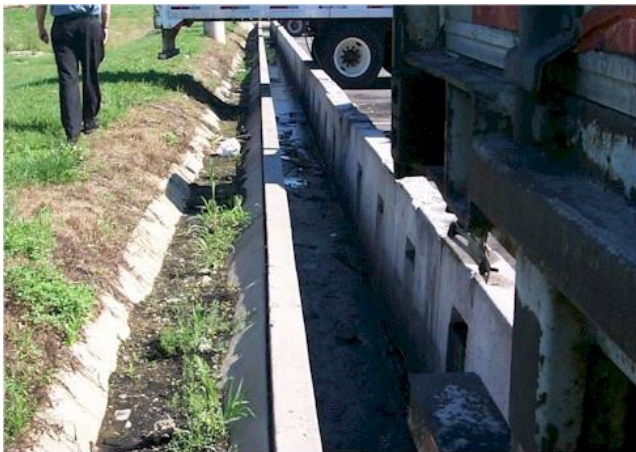
Figure 9-16. Perimeter trench drain.
